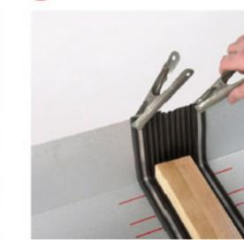
Clamp the Expansion Strip Joint into position and press into corners of the box gutter with square object (e.g. piece of wood).
