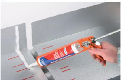
Apply a neutral cure silicone bead along the line of rivet holes on both box gutters.
