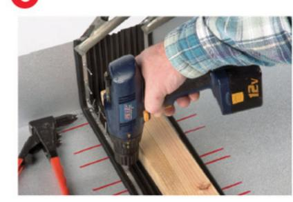
Hold the Expansion Strip Joint in place whilst drilling rivet holes. Place rivets temporarily in position to stop flashing moving whilst drilling additional holes.
