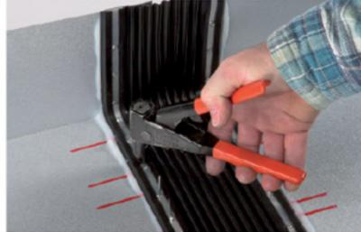
Pop rivet the Expansion Strip Joint in place and smooth over the Silicone to complete installation.
