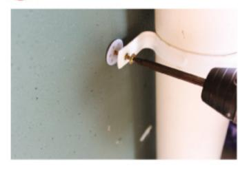
Place the clip or bracket over the Styroscrew anchor and secure with the metal screw you have selected.
