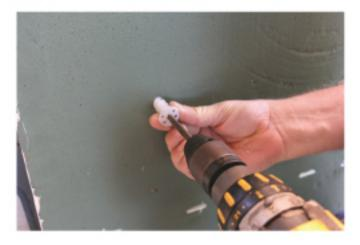
Using a Phillips driver bit, screw the Styroscrew anchor into the board until the flange is firmly against the board. 3
