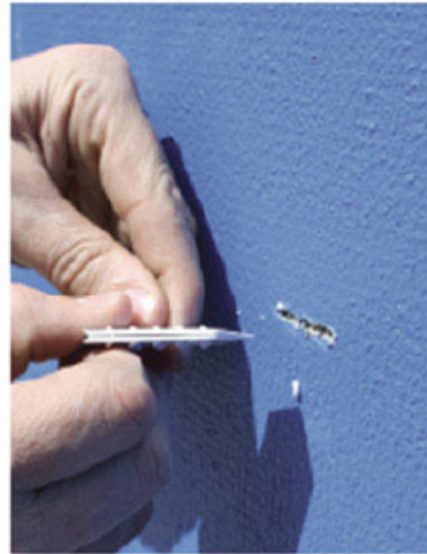
Insert the Styrowedge into the slot in the wall.
