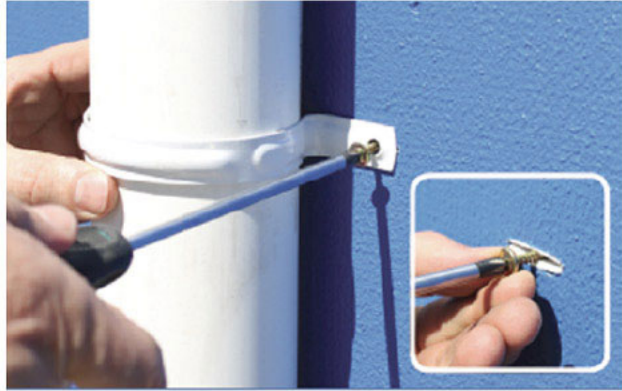
Place the downpipe and clip in position on the wall. Insert an 8-12 gauge screw into the Styrowedge and tighten into place.
