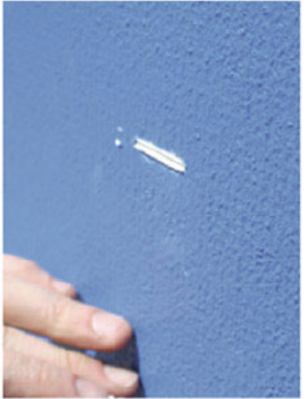
Ensure the Styrowedge is flush with the finish of the wall.
