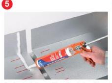
Apply a neutral cure silicone bead along the line of rivet holes on both box gutters.
