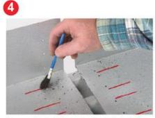
Remove the flashing and pull out rivets to brush away any metal swarf.
