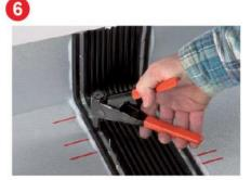
Pop rivet the Expansion Strip Joint in place and smooth over the Silicone to complete installation.
