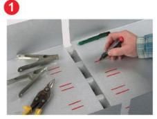
Mark the position of the support tray alleys on the gutter to allow for rivet installation clearance.
